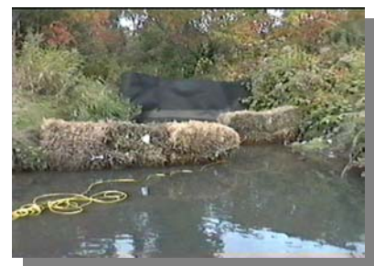
Water run-off from tunnel feeds creek that needed protecting.
