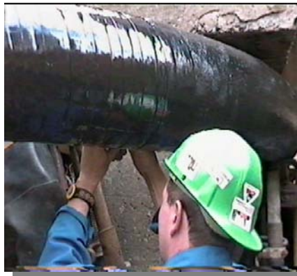
6" wide KemaSeries60 was used with a 50% overlap.
