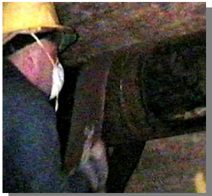
Underground—where pipe cleaning with aluminum oxide paper is the norm.
