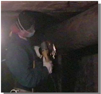
Power wire brush cleaning in preparation for liquid primer application.
