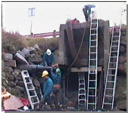
Safety practices included escape ladders, harnesses and supplemental air supply.
