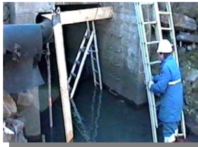
Looking down at water-filled tunnel entrance.
